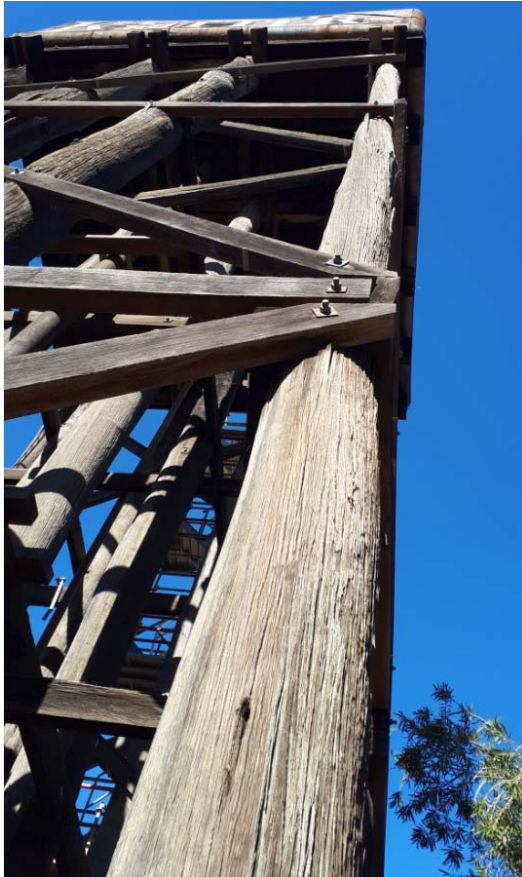
Figure 9 Tank Timber Columns
