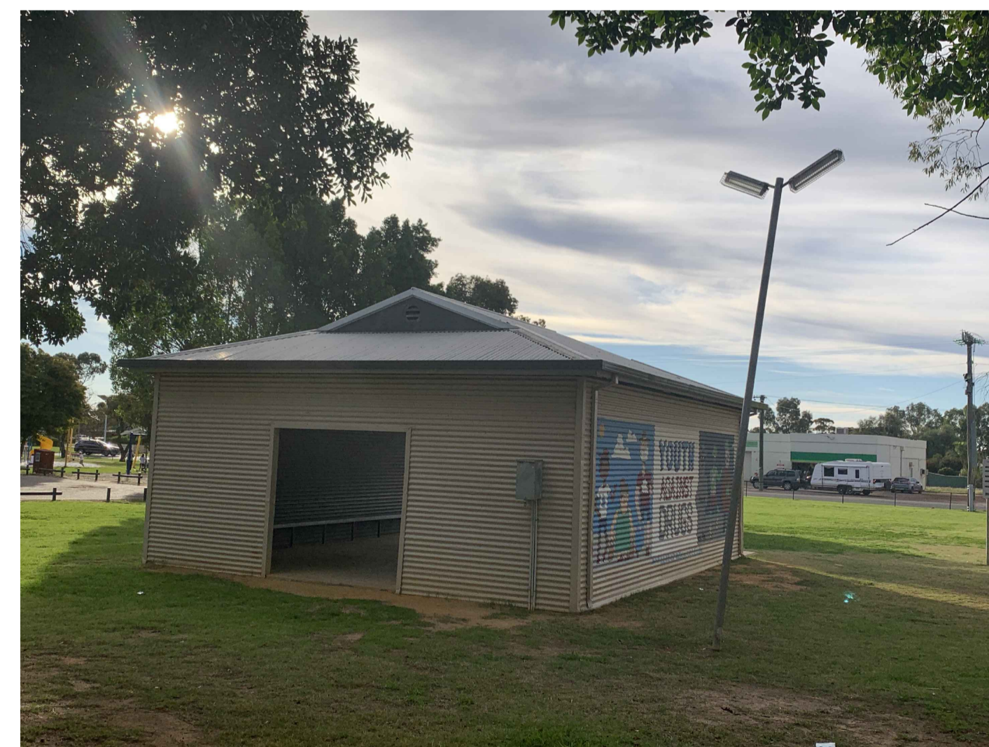
07 SOUTHERN ELEVATION SITE PHOTOGRAPH
