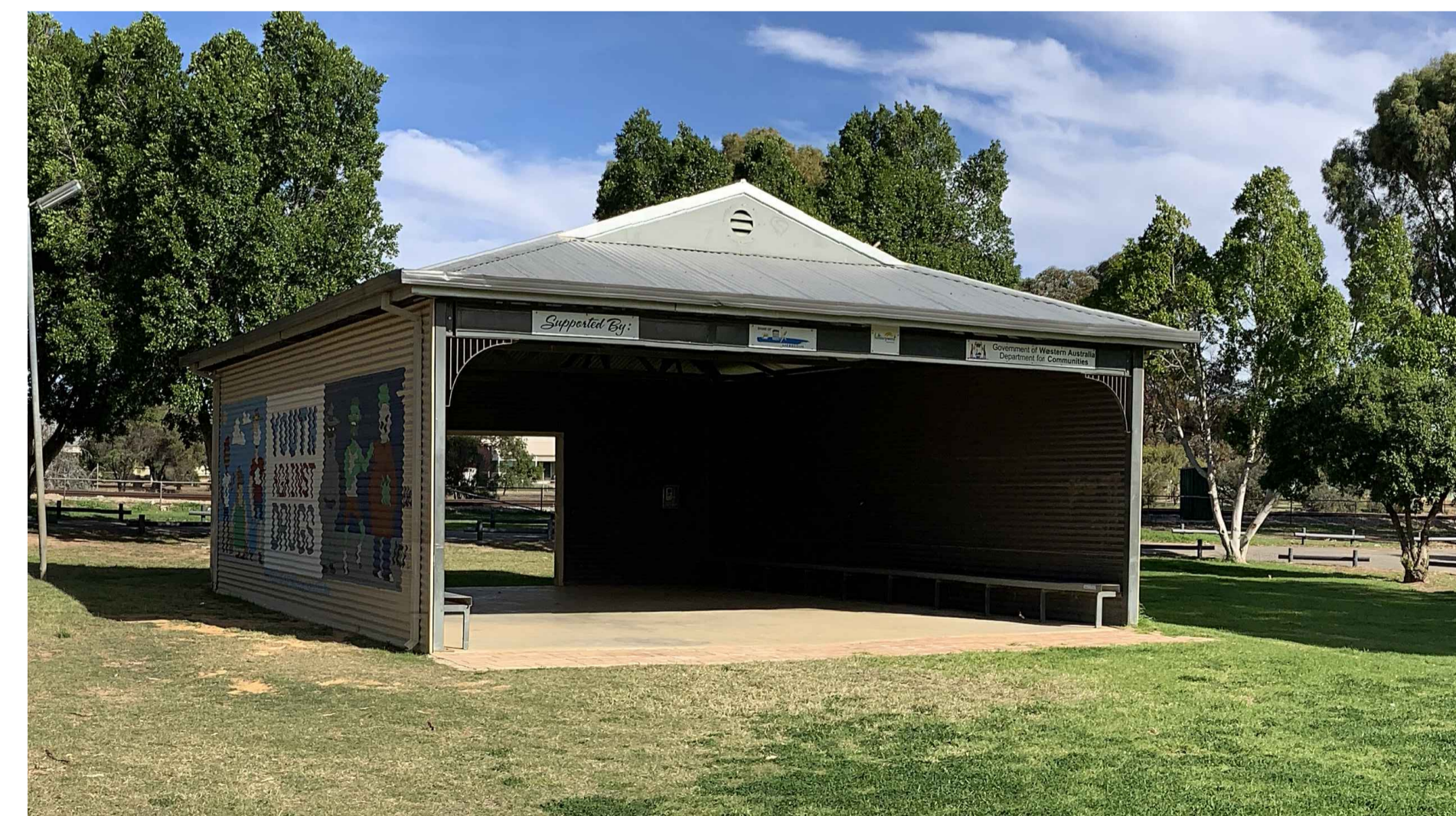
06 NORTHERN ELEVATION SITE PHOTOGRAPH
